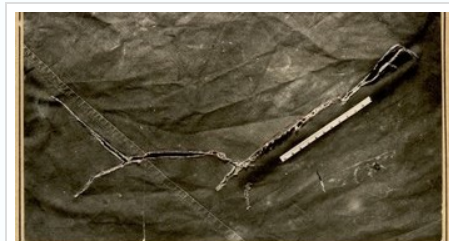
Photo N.4 General view of damages type 1
