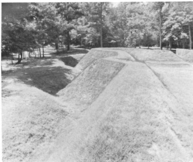
FIGURE 26—Stabilization of the fort
